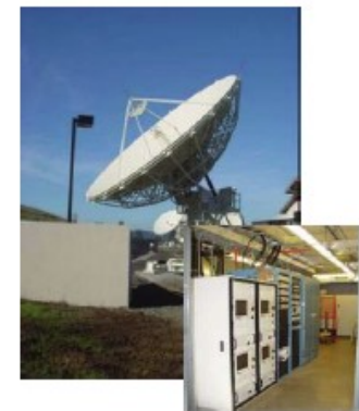
4 Ground Earth Stations
